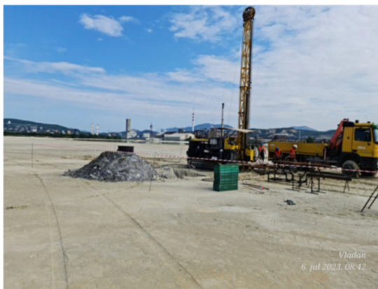
Figure 15: Field work at the Old Bor flotation tailing pond (Field I and Field II).
